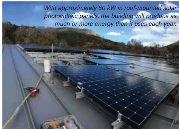
With approximately 80 kW in roof-mounted solar photovoltaic panels, the building will produce as much or more energy than it uses each year.
